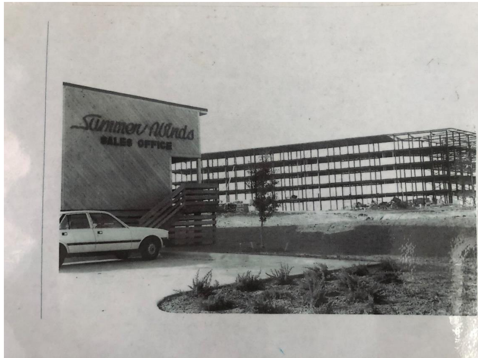
Summer Winds "A" building under construction.
